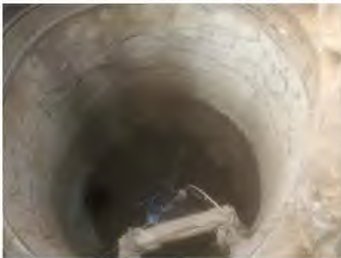
Manhole at 636 Showing Relining and Plugging of Catch Basin Lines
