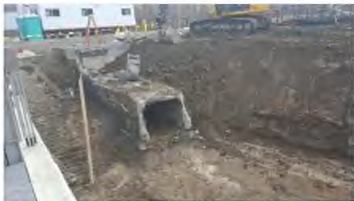
Influent Structure #2 with Hand Operators and Stairs Removed
